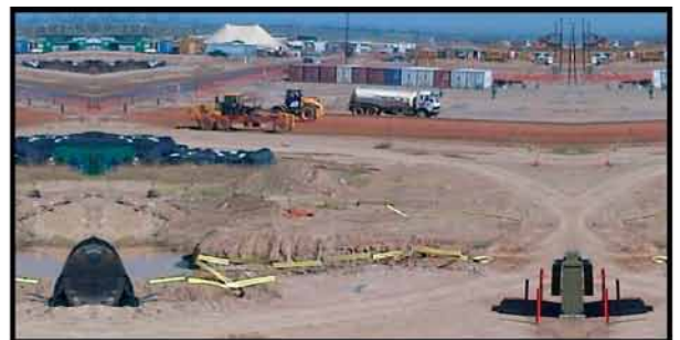
KUSILE POWER STATION: CONCOR VENT CONSTRUCTION AREA
