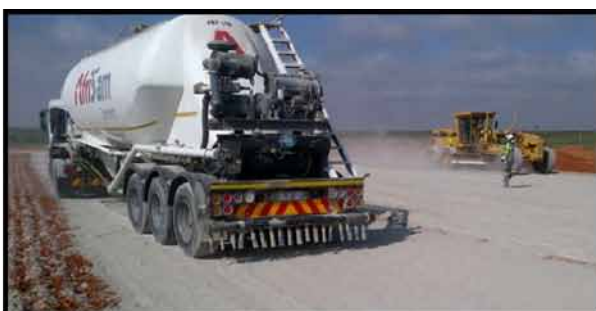
KHUTALA COLLIERY: CEMENT STABILIZATION OF SUBSTATION PLATFORM LAYER WORKS
