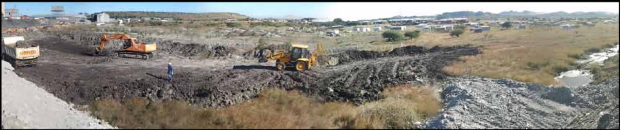
EASTERN PLATINUM: SETTLING PONDS CONSTRUCTION
