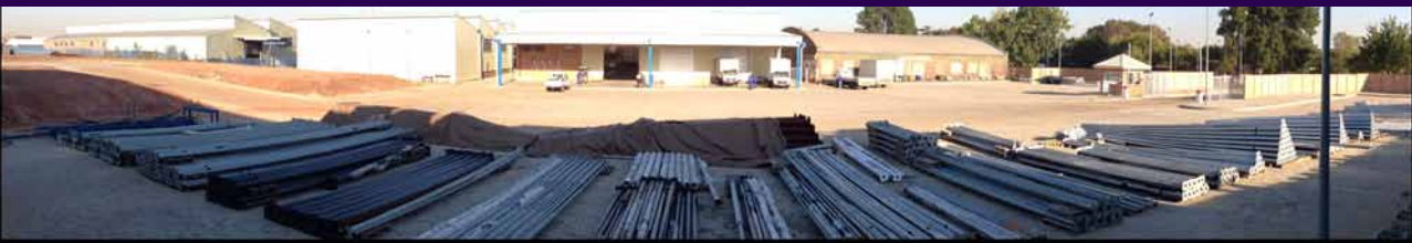
CANDELA WAREHOUSE: BULK EARTHWORKS AND EXTERNAL WORKS
