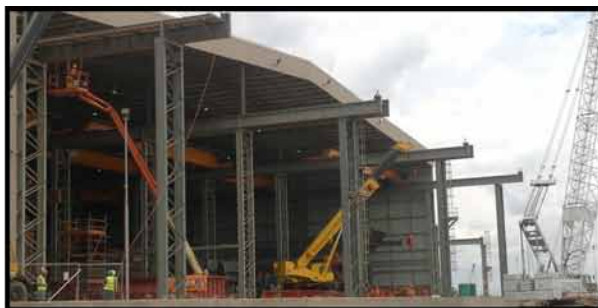
KUSILE POWER STATION: WORKSHOP GANTRY EXTENSION
