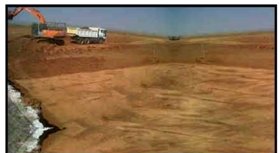
KHUTALA COLLIERY: BOX CUT FOR SUBSTATION PLATFORM
